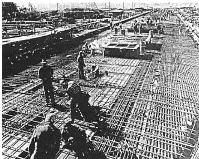
Figure # 3 —Construction of lightweight concrete ship—World War II
